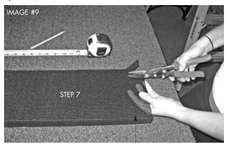
NOTCH OUT SPACE FOR WALL ATTACHED BRACKETS
